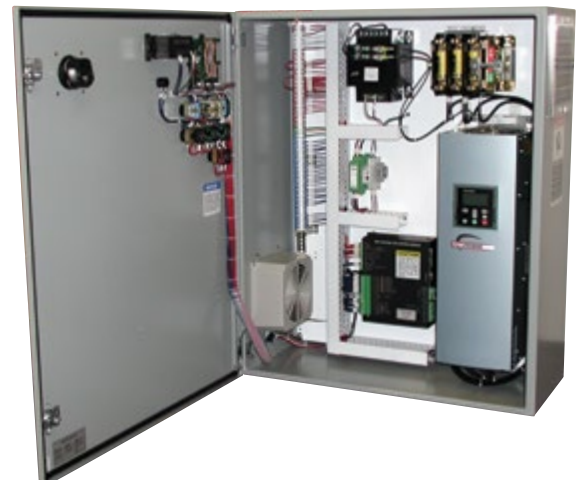
Special Control With Enclosure Door Open Showing SSC1500 Control, Variable Frequency Drive, and Other User-Requested Components
